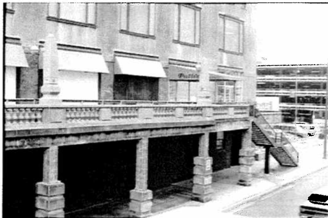
The building's west elevation was designed (left) so that another structure could be built behind it without blocking the light of most offices. The Grand Avenue facade (right) includes lower-level loading docks, sheltered by a classical-style balustrade.
